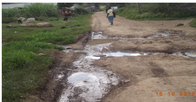
Most Rural access roads in the county are impassable
